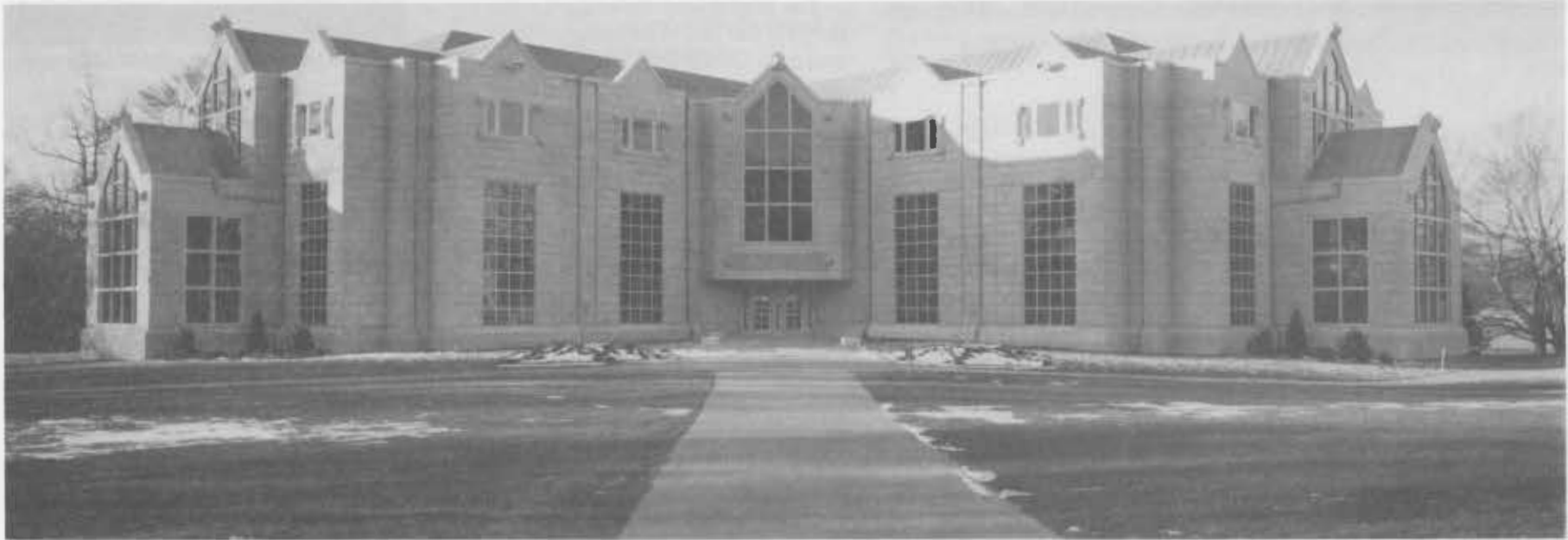
The new College Library displays its rock-face granite exterior with the peaks of its copper roof thrust toward the winter sky. Construction continues on the interior of the technologically advanced facility which is anticipated to open this year.
