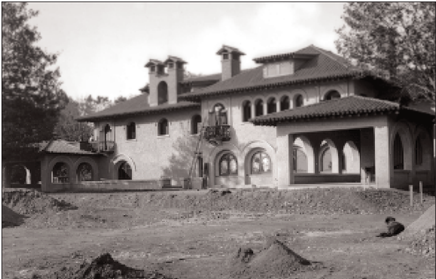
Mason House under construction, 1902
